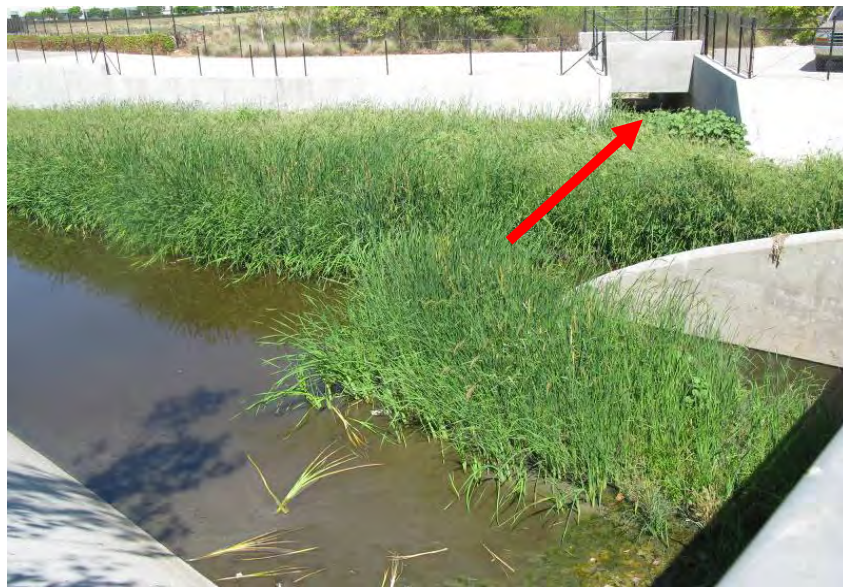
Site ICSC showing the reinforced concrete box entrance (red arrow) that connected the San Diego Creek to the channelized Serrano Creek, which showed standing water.
