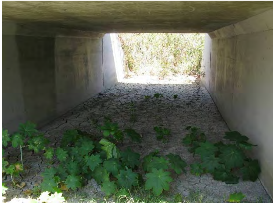
Site ICSC on the northeast side of Irvine Center Drive showing the inside of the reinforced concrete box that connected the San Diego Creek to the southeast channelized wall of Serrano Creek.
